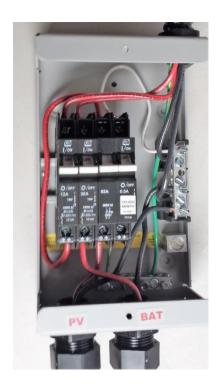
**Important:** The circuit breaker torque value is 20 inch-pounds (2.3NM). You should tighten to this specification during installation and again one hour after the installation is powered up. Do not omit the second tightening! A loose wire can cause arcing, melting of bus bars and fire.
