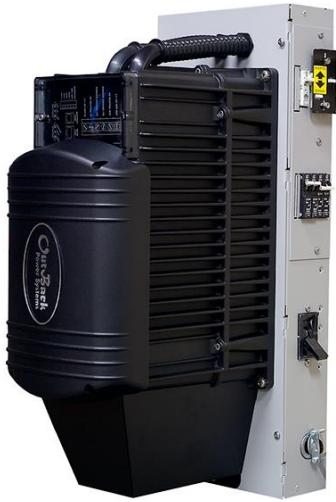
OutBack E-Panel as installed (narrow)
