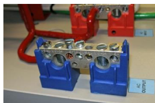
Replace the Busbar and press into place
