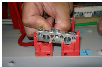
Finish removing the terminal block
